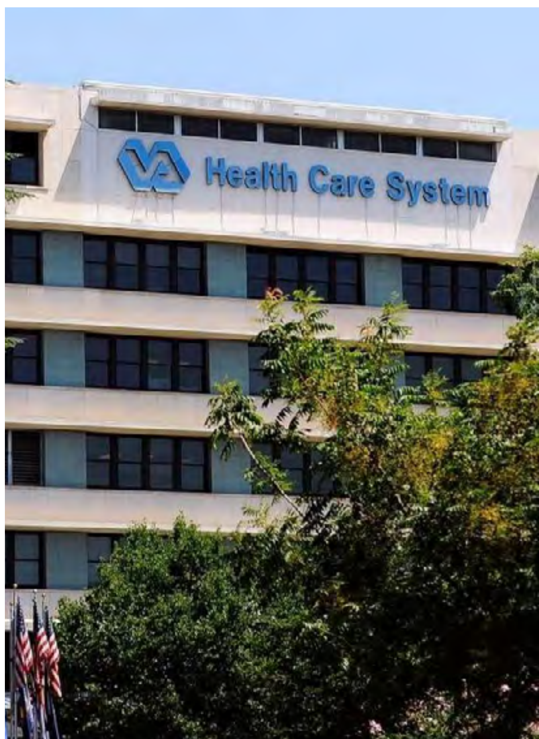
VA HOSPITAL MULTIPLE PROJECTS Fresno, CA
